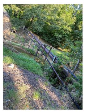
Original steel pipe suspended over the canal
